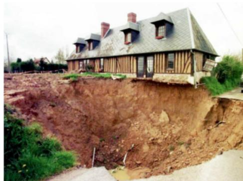
well blocked by rocks (view from inside the underground cavity) - Collapse under a house.
